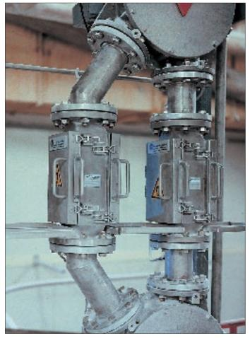
To ensure that the continuous process is not interrupted, a double outer system is used in this application
